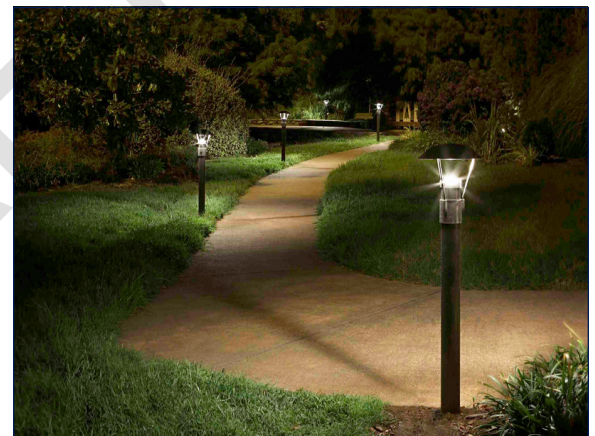
Bollard lights can effectively light a trail corridor without spilling over into the neighboring environments.
