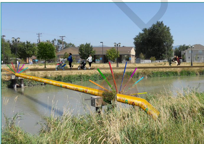
A trail along the Surplus Canal would provide more recreational opportunities and open up the potential to incorporate public artwork in conjunction with Salt Lake County and the community.
